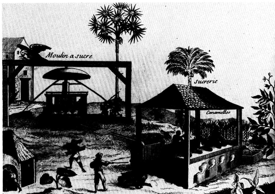
FIG. 4—A three-cylinder mill in a West Indian sugar factory. Source: Pierre Pomet: *Histoire Générale des Drogues* (J.-B. Loyson, Paris, 1694), p. 94. (Reproduced by permission of the British Library Board.)
